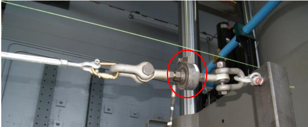
Figure 23 – Load cell (44.5 kN) for measuring cable tension (taken from Leclerc and Tremblay, 2015)
