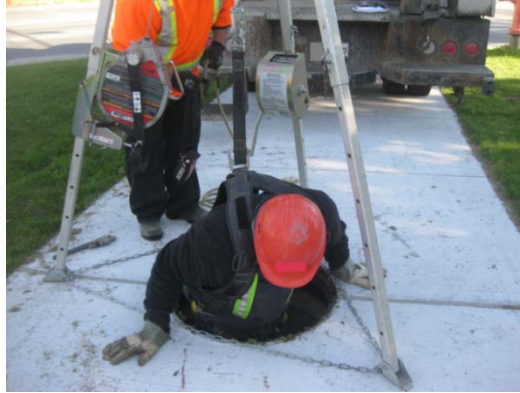
Figure 6 – Tripod and winches for fall protection and rescue without entry; wearing of a Class A harness
