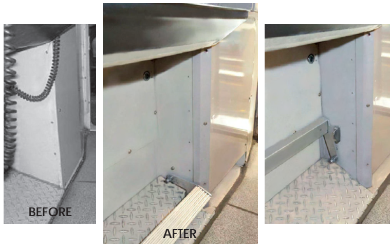
The area beneath the control console before and after the modifications.
