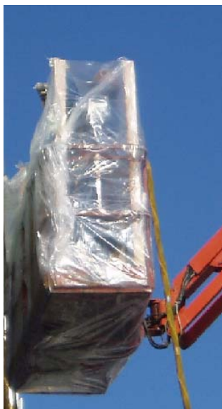
Figure 4: Non-compliant shelter on a motorized elevating platform
