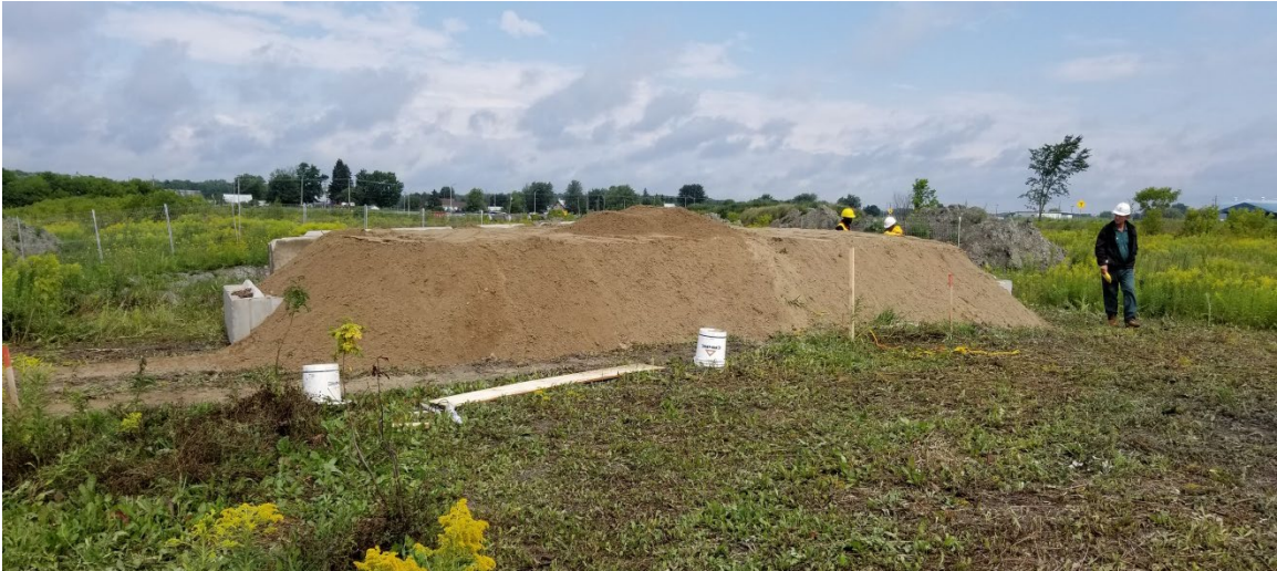
Figure 26. Loading of trench A2 with concrete blocks and sand.
