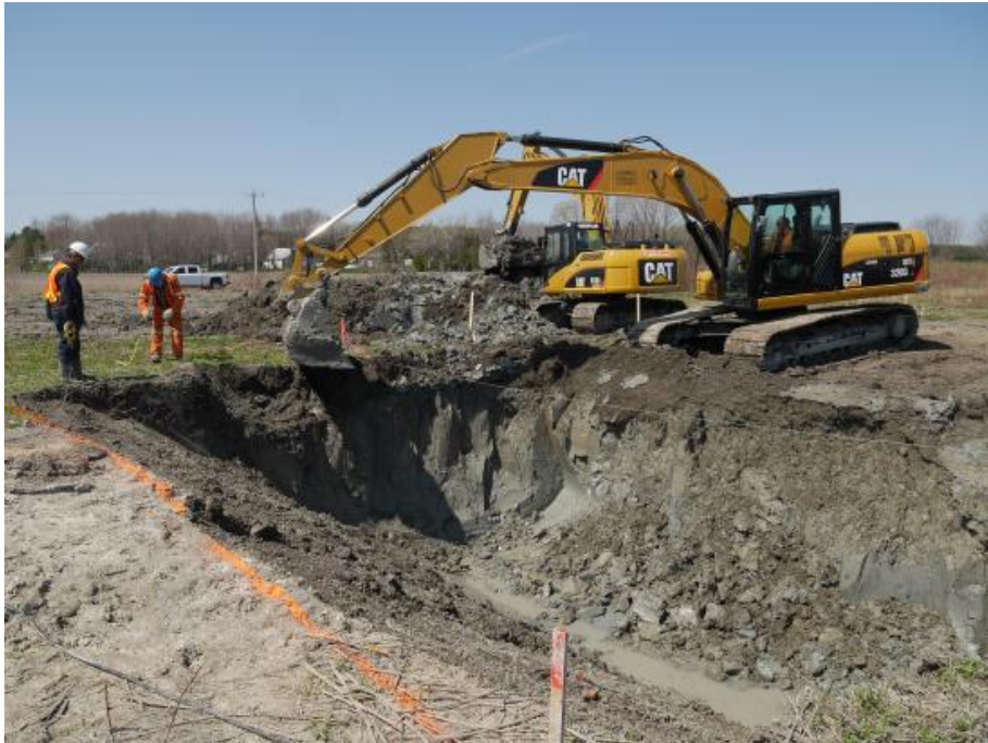
Figure 20. Digging of trench A2 with Caterpillar 315 and Caterpillar 320 excavators.
