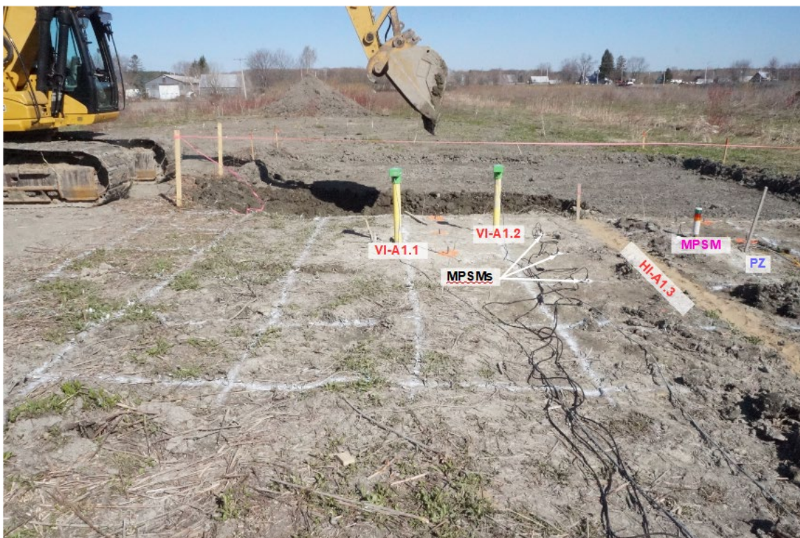
Figure 16. Excavation of trench A1.
