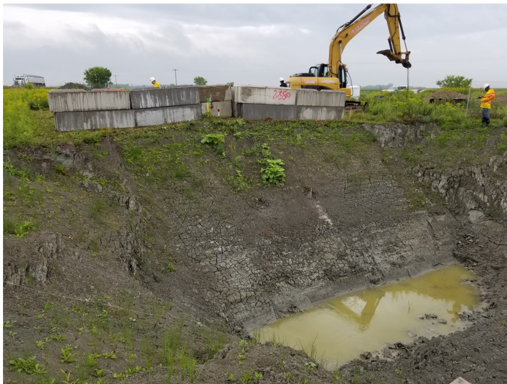
Figure 23. Loading of trench A2 with concrete blocks.
