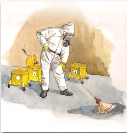
Figure 2: Wet clean-up technique with three pails
