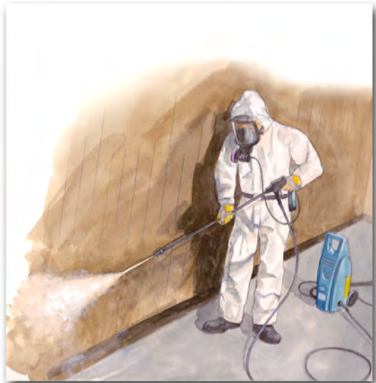
Figure 3: Washing technique with low-pressure water jets
