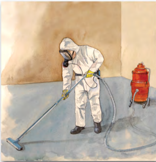
Figure 1: Vacuum cleaning using a vacuum equipped with a HEPA filter
