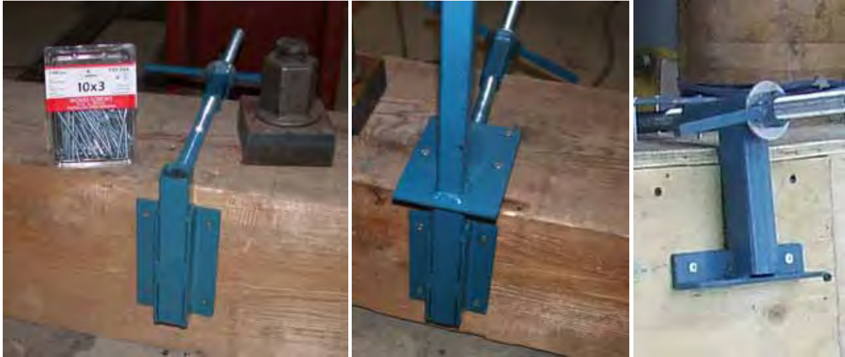
Figure F-5 – Ancrage des garde-corps Alcor.
