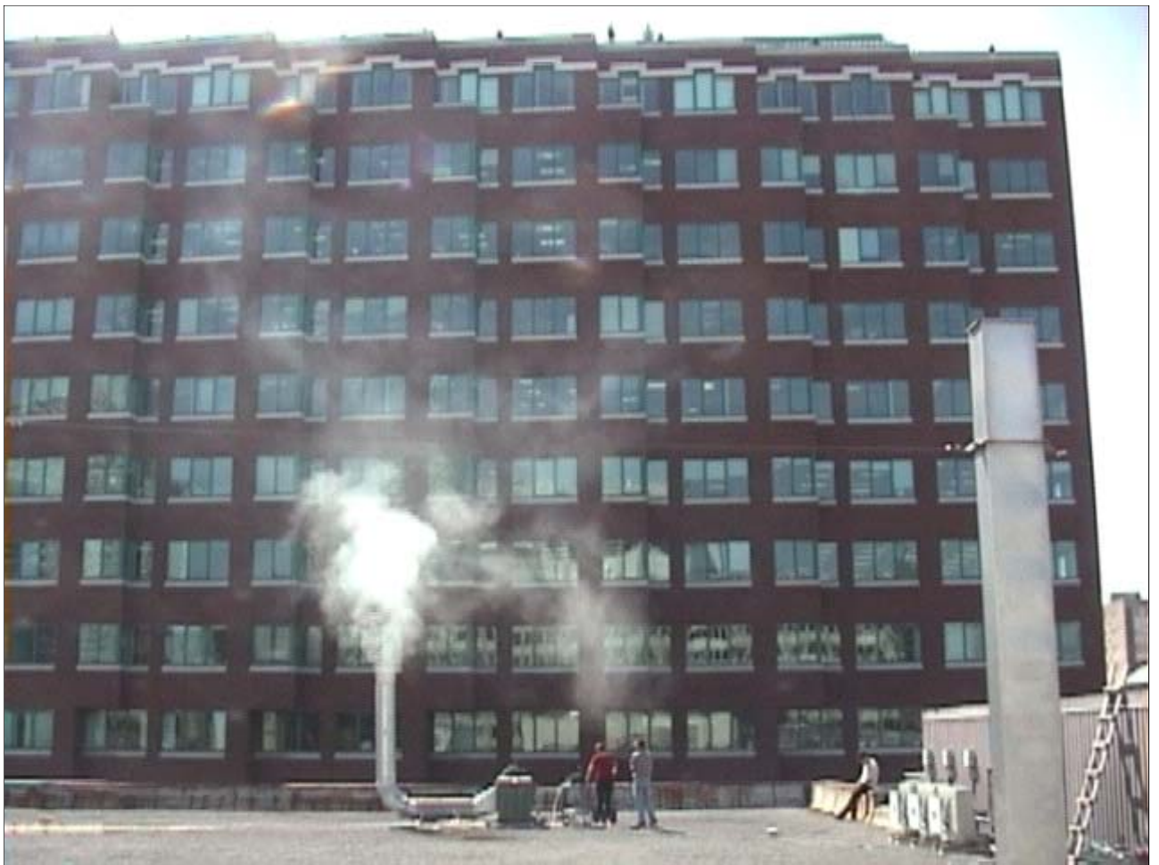
Figure 5.31 Smoke visualization test for September-06-02 hour 2 field test: Stack location 3
