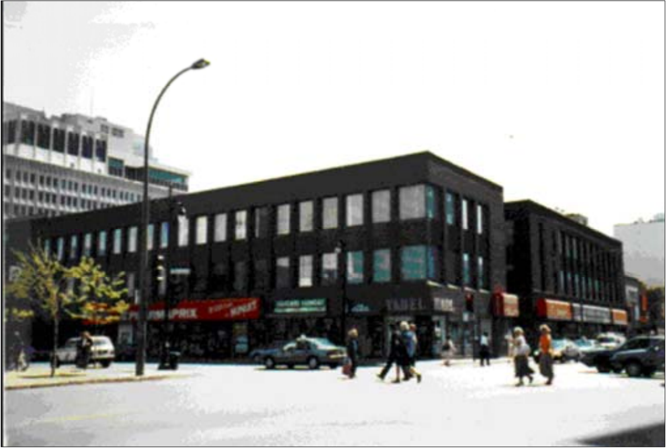
Figure 4.1 BE building, Centre for Building Studies, Concordia University, Montreal viewed from west
